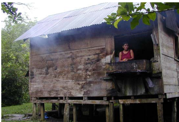
The STIBRAWPA Group's Yorkin Headquarters
